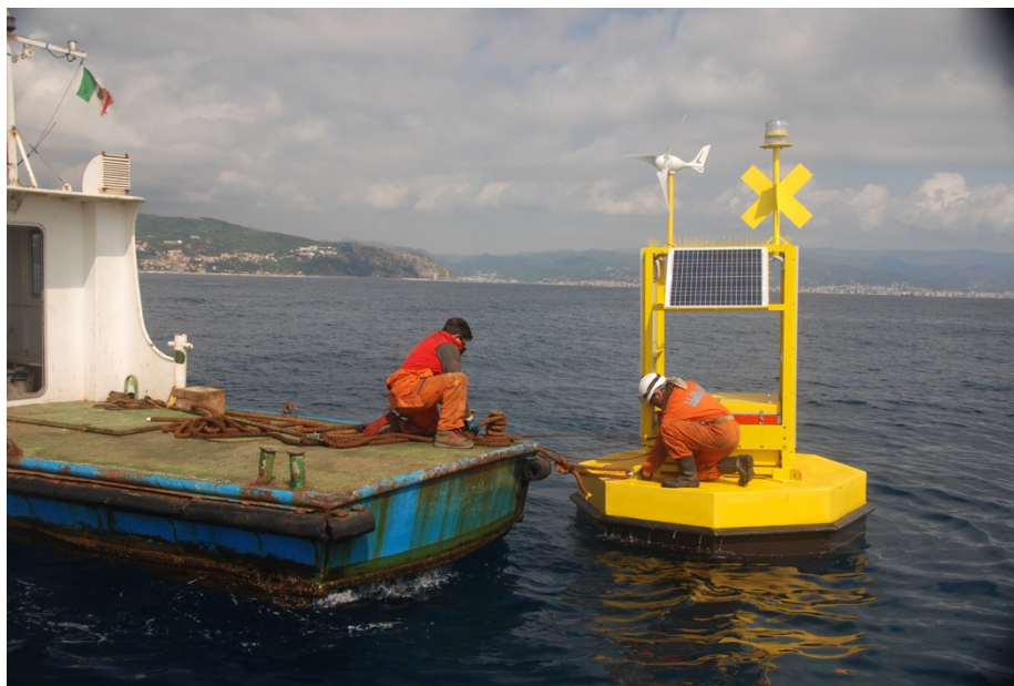
Figure 18: Deployment of a main buoy
